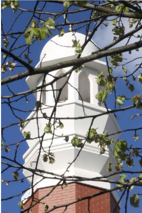
Manchester Central Mosque
